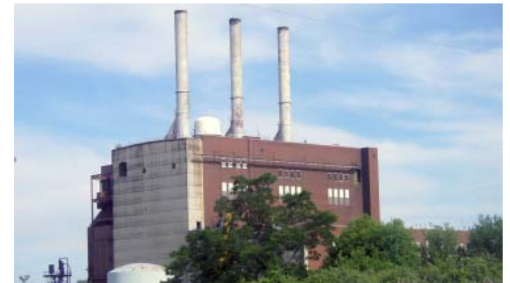
Consumers Power Plant
