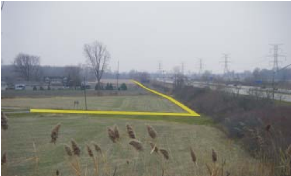
Potential Alignment of Non-motorized Trail Along I-75. View Looks South From Gaynier Rd.
