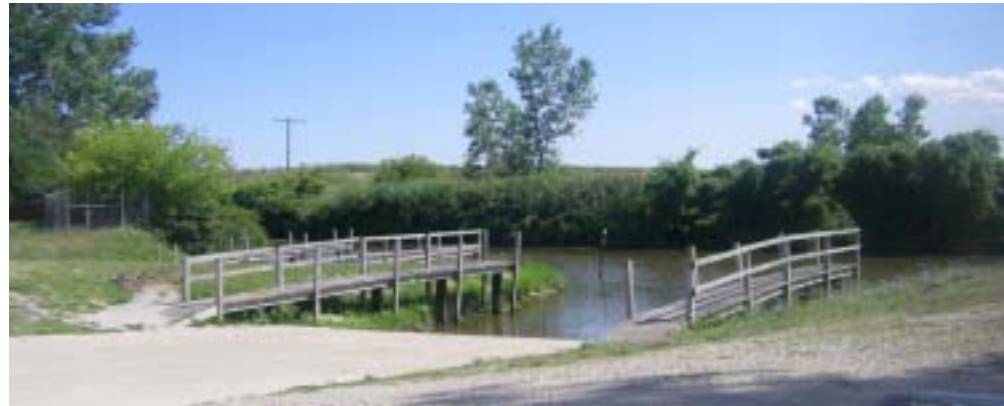
Existing Municipal Boat Ramp
