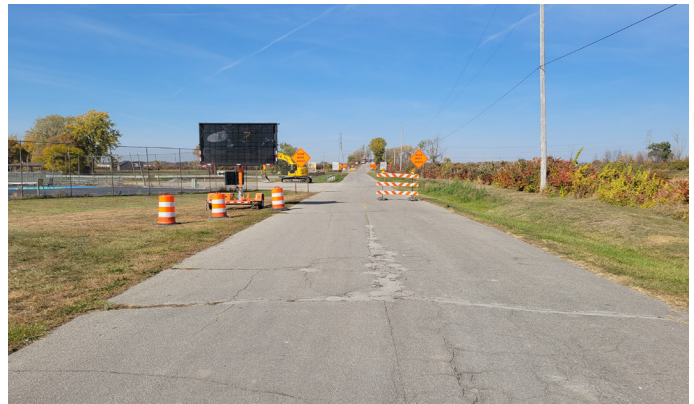
Gaynier Road - Looking northwest from Harold Drive
