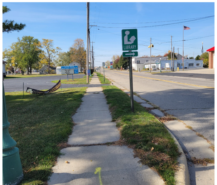
Luna Pier Road - Sidewalk along south side of road
