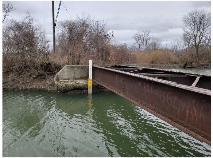
Old interurban trolley line bridge over Whitewood Creek
