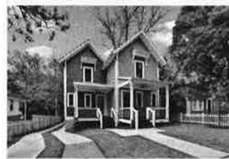
Duplex (2-unit structure)
